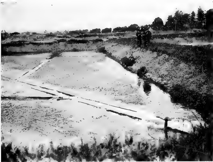
Fig. 47.—Sand filter of a sewage disposal plant.
